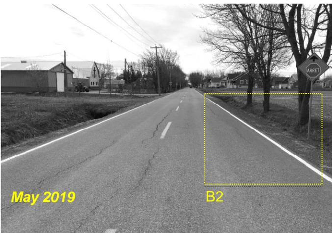
**Figure 9. Isolated Longitudinal Cracks Observed on the Trial Section in May 2019 Field Follow-up**
