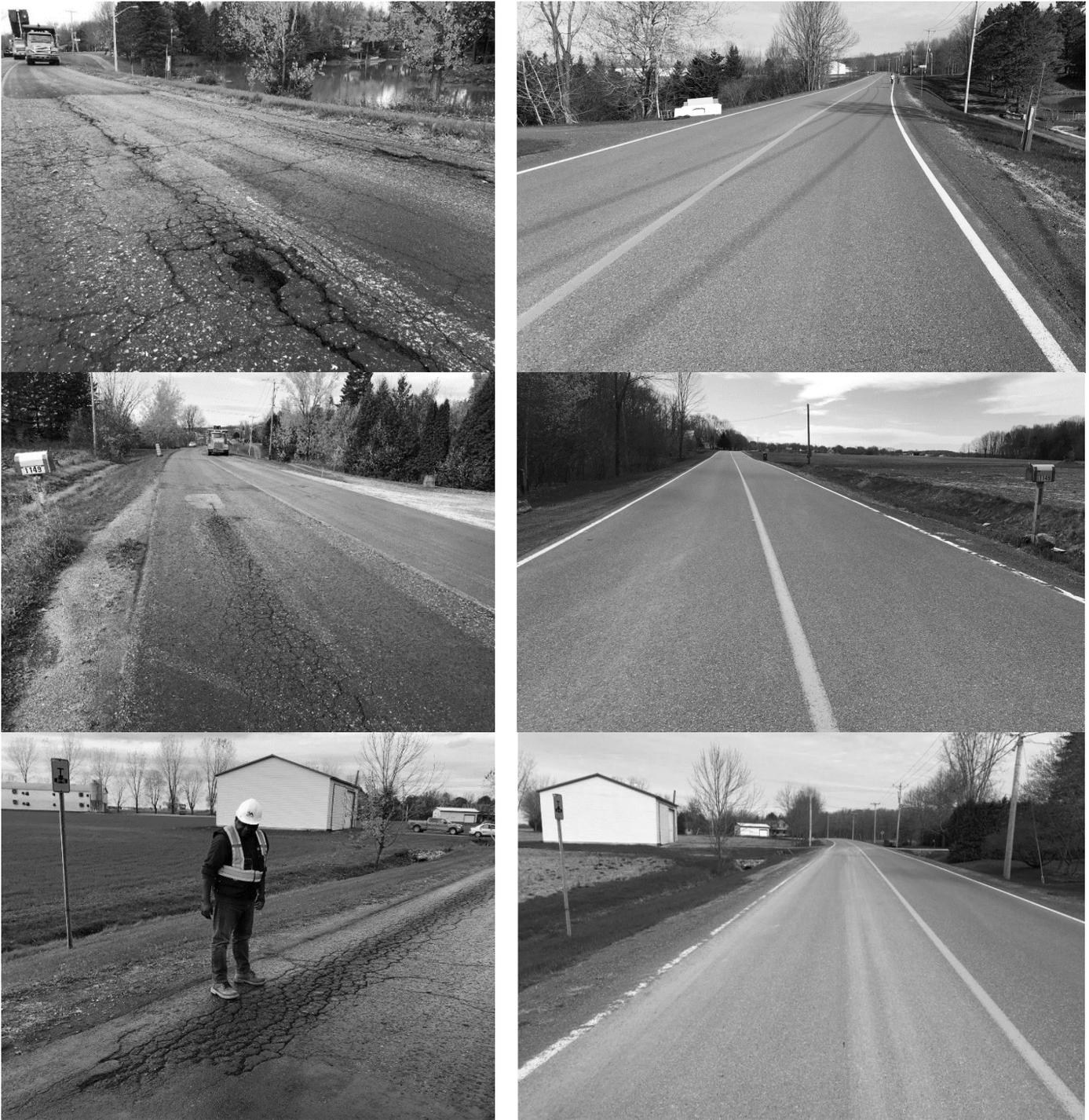
**Figure 7. Distresses Documented in October 2017 Prior to Placement of Enrobés Flexibles Municipaux (EFM) Overlay (Left Column) and Same Locations in May 2019 (Right Column)**
