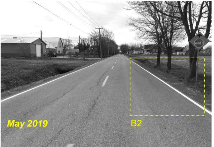
**Figure 9. Isolated Longitudinal Cracks Observed on the Trial Section in May 2019 Field Follow-up**
