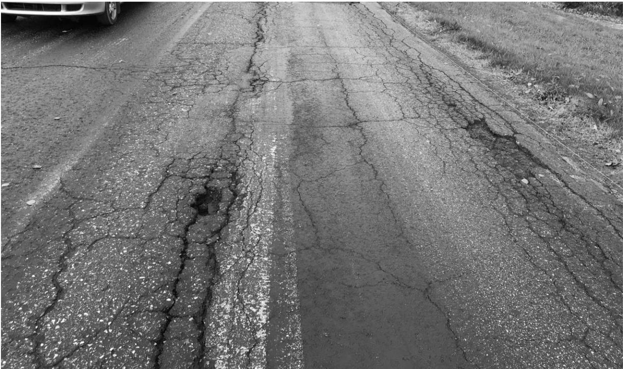
**Figure 1. An Example of Road Candidate to Receive Enrobés Flexibles Municipaux (EFM) Overlay**
