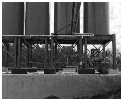
(b) A small tonnage of the mix was produced to check discharge after the drum and silo. This was also to clean the belts and ensure the designated silo is free of contamination
