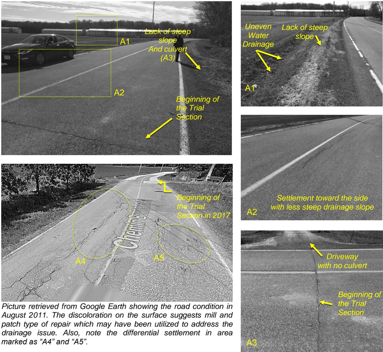
Picture retrieved from Google Earth showing the road condition in August 2011. The discoloration on the surface suggests mill and patch type of repair which may have been utilized to address the drainage issue. Also, note the differential settlement in area marked as “A4” and “A5”.
